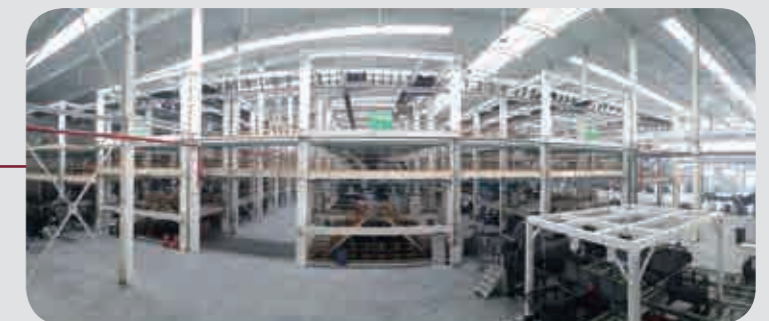
Threading, Air Pressure Test, and Anti-rust Treatment
